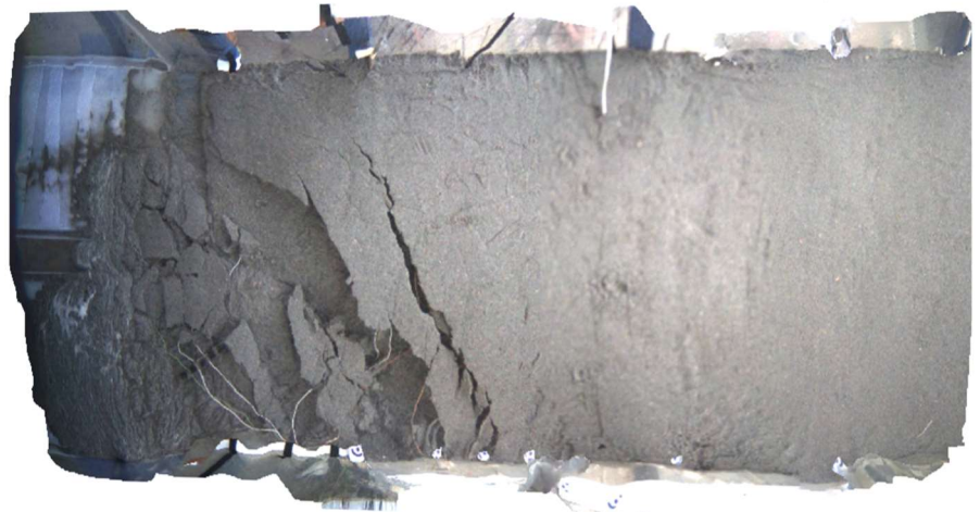
Fig.71. 90 degrees inclined Orthophoto of
