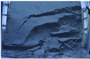
Front Camera, Fracture 7
