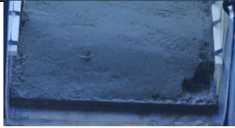
Front Camera, Fracture 1
